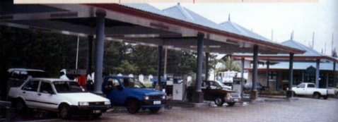
New Petrol Station - Roche Calman
